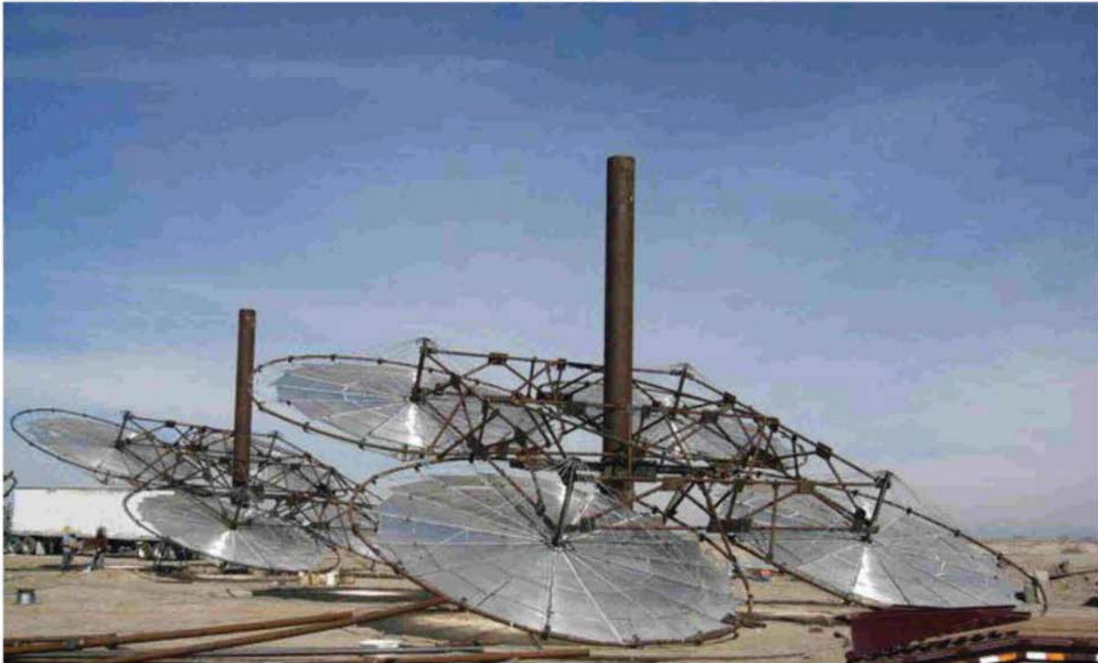
(Figure 6: IAUS solar field under construction)
