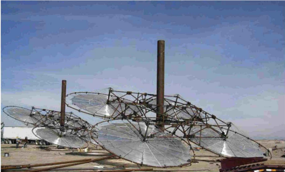
(Figure 6: IAUS solar field under construction)
