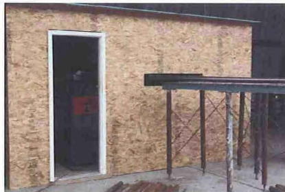
Manufacturing: Installed pipe-bender with insulated housing.
