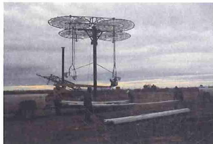
Installation: Delivering insulated pipes from the manufacturing plant.
