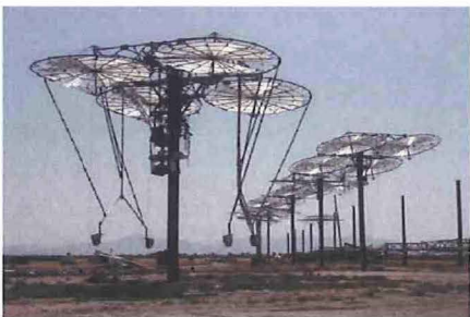
Installation: Starting to add the heat concentrators.
