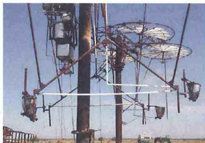
Installation: Tower with the new heat collectors, heat concentrators and new insulated white pipes.
