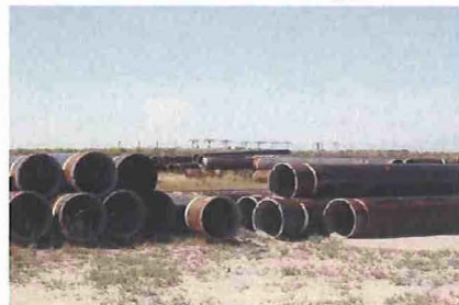
Installation: More steel delivered to the solar site.
