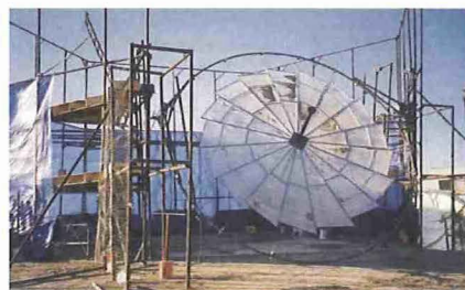
Second Tower Design: A two-disc solar tower concept was constructed with idea of lowering construction costs over the single-disc concept.
