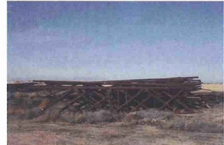
Field Construction: Manufactured components being delivered and stacked.
