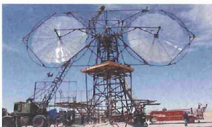
Second Tower Design: The two-disc tower concept required a gantry crane. Today, the disc-assembly and hydraulic tracking systems are installed at ground level and raised as a complete unit saving time and money.
