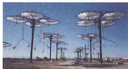
Installation: Our R&D towers being converted to commercial spec units.
