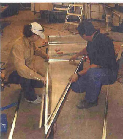
R&D Fabrication: Here are workers assembling the first solar-lens frame. Currently, we are on our 5th solar-frame design. The current design can withstand winds up to 100 mph.
