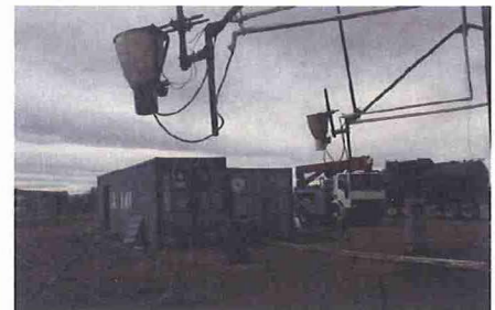
Installation: The biomass container is on the left and the solar energy container on the right.
