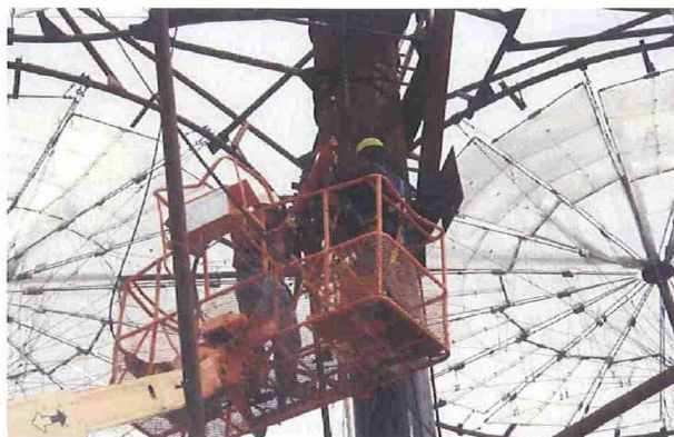
Installing the dual-axis tracking system.
