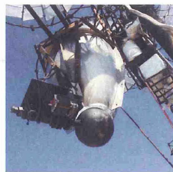
Installation: Close up of the newly installed gear-driven heat collectors or "magic ball".
