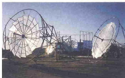
First Solar Tower Concept: Construction on the original single-disc tower design.
