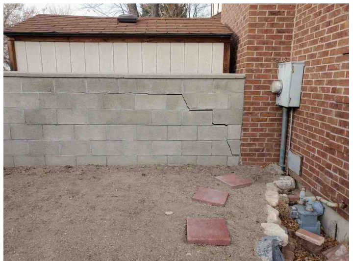
Concrete Block Fence
